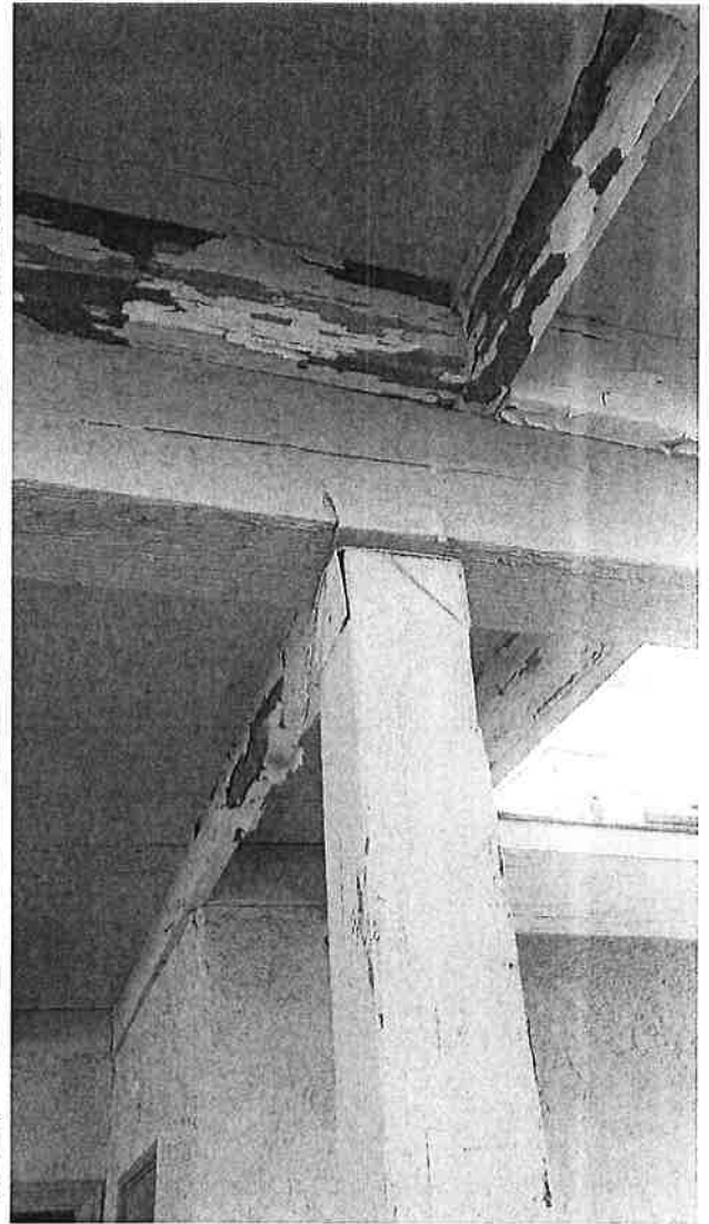
Photo 4 – Closeup of Column Connection.
